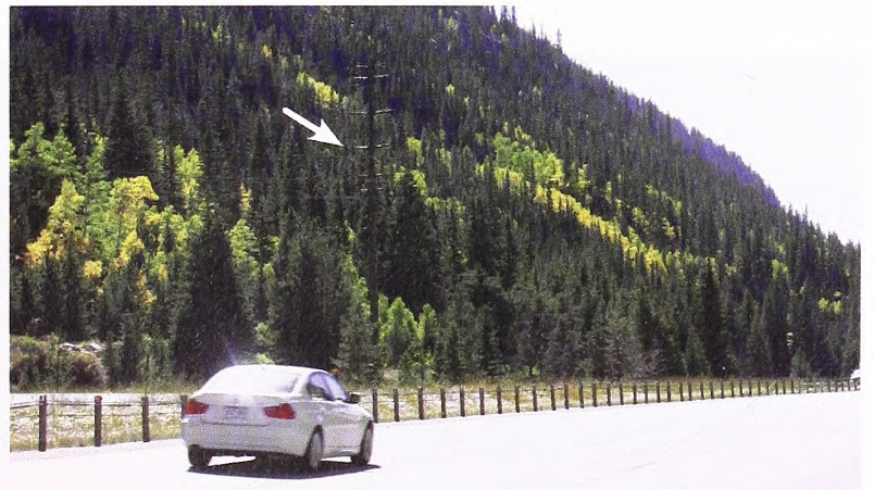
Transmission power line that was factory painted with a single color and installed circa 1976.
